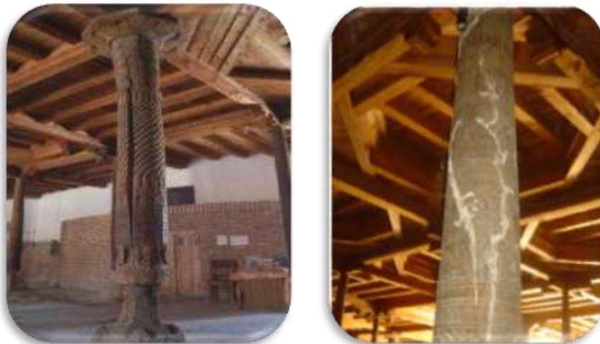
Figure 2. The wooden columns affected by termites1. Mechanical damage (bent, tilted, cracked, and so on) 2. Biological damage (termites)
